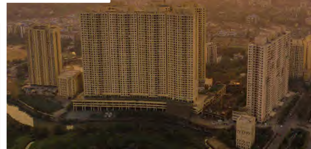
→ Shot at location - Rustomjee Urbania
