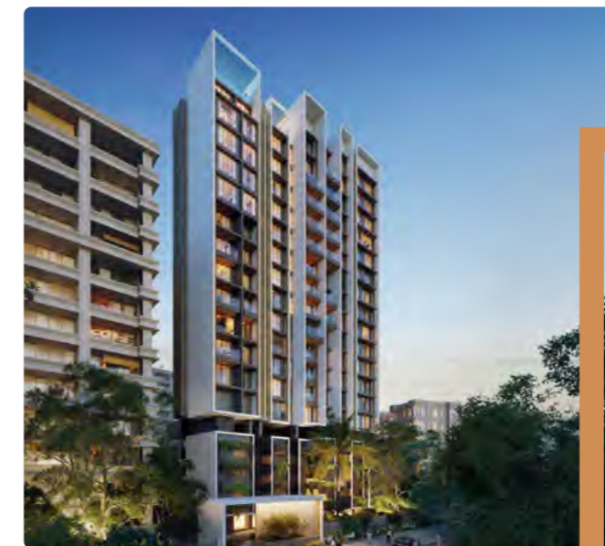
↑ Rustomjee Parishram PALI HILL, BANDRA → SP
